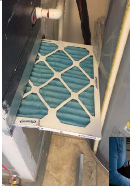
"Filter Lock" uses magnets to seal access
