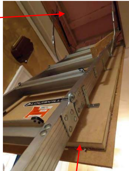
Insulation in stairs door
