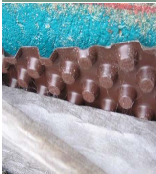
Spray on water-proofing plus drainage board
