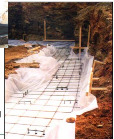
Plastic wrapped beneath footing
