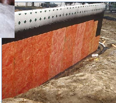
Spray on water-proofing plus drainage board
