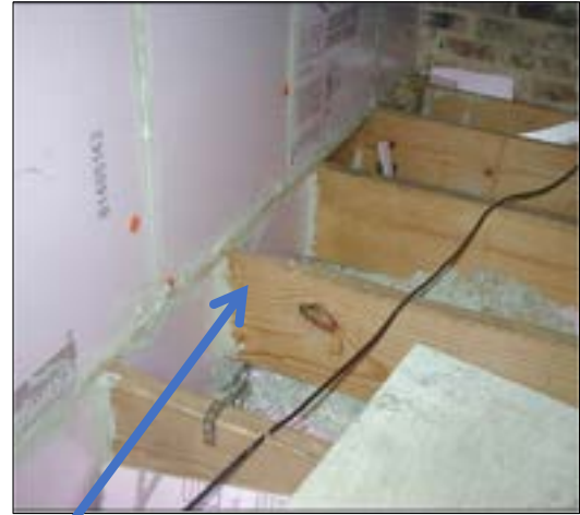
Install Kneewall blocking
