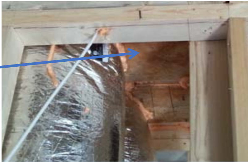
Chase capped and sealed around duct
