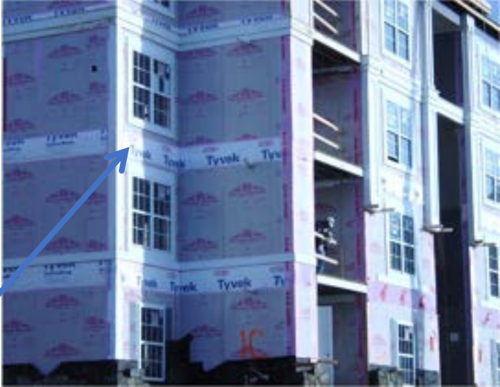
Sheathing sealed and sealed housewrap at band
