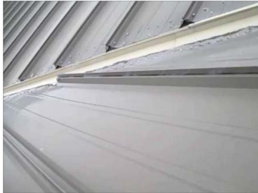
Roof above shims
